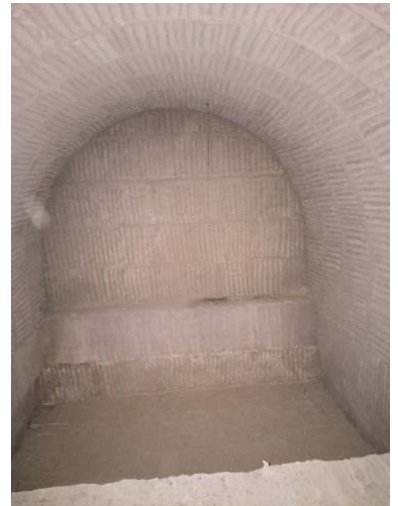
Inside combustion chamber
